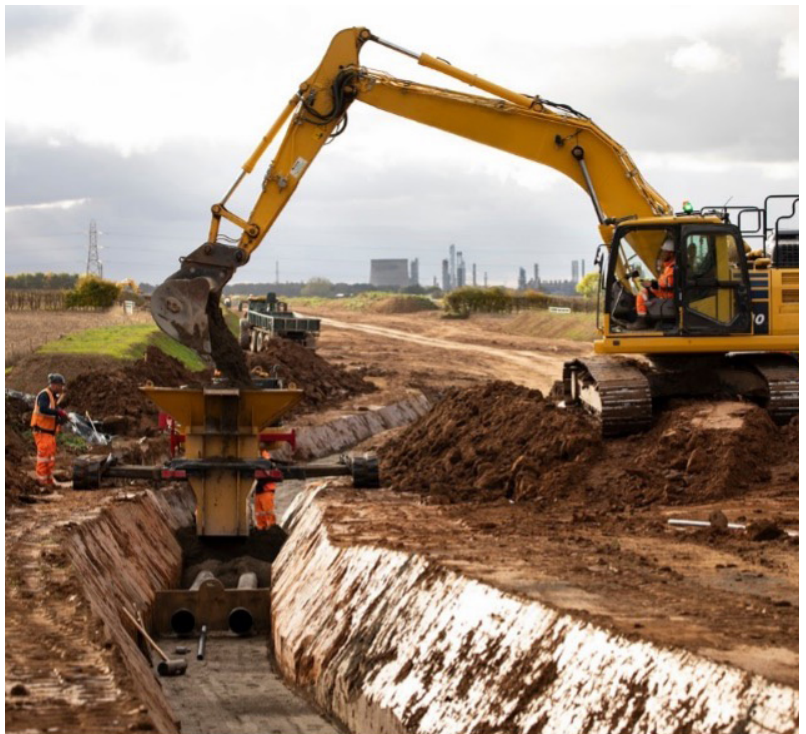
Backfilling a trench with cable ducts laid (Sofia Offshore Wind Farm)
